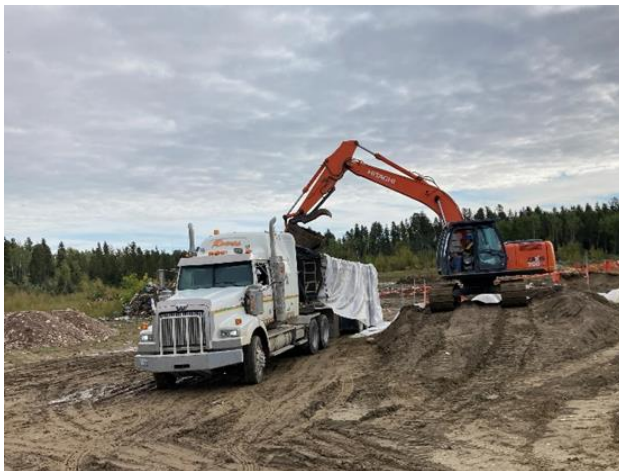
Loading material into lined truck bed
