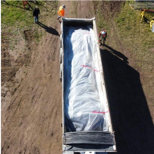
6 mm poly sheeting lines trailer, encases material
