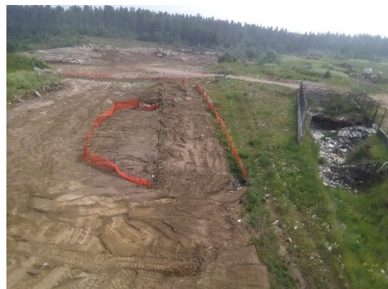
Fort Smith landfill cells grubbed to expose cover material
