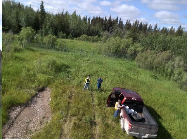
Project staging area for excavated soils and loadout
