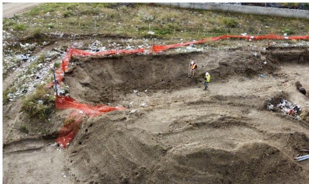
Technicians conducting verification gamma scans
