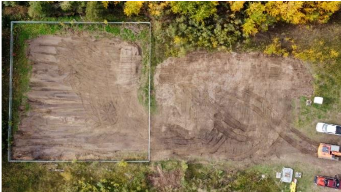
NTR Phase 1 - Fort Fitzgerald Mound - Temporary Storage Area
