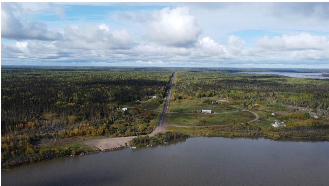
Fort Fitzgerald TSA removal/restoration complete - September 2021
