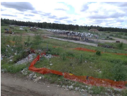
Fort Smith Landfill cells – Day 1
