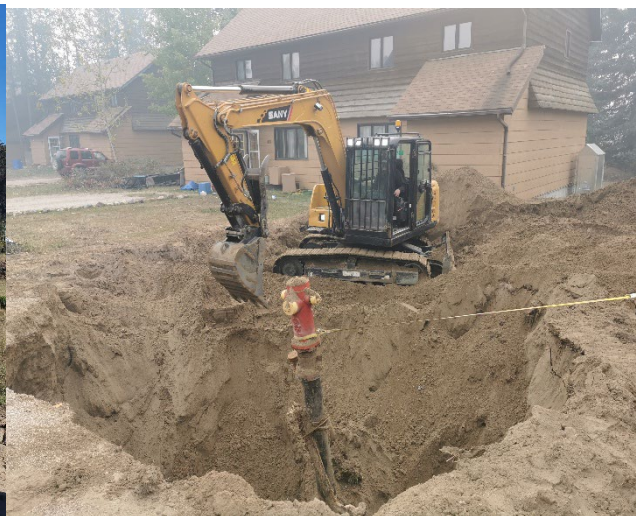
Hydrant replacement in the coop
