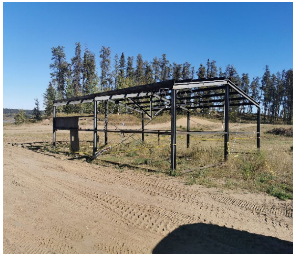
Steel Frame to be moved to the landfill
