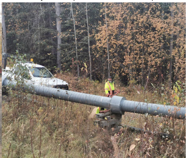
Working on the raw water transmission line.
