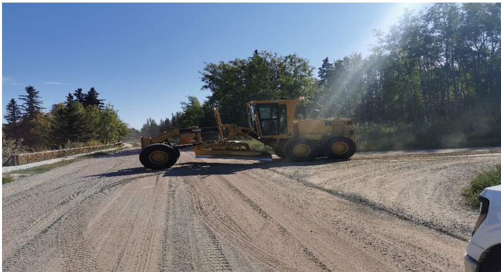
Grader at work stress testing while working on roads
