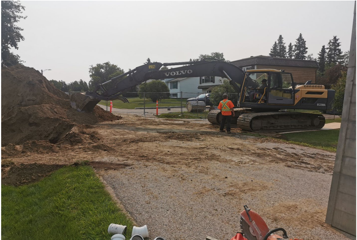
Sewer repairs being completed
