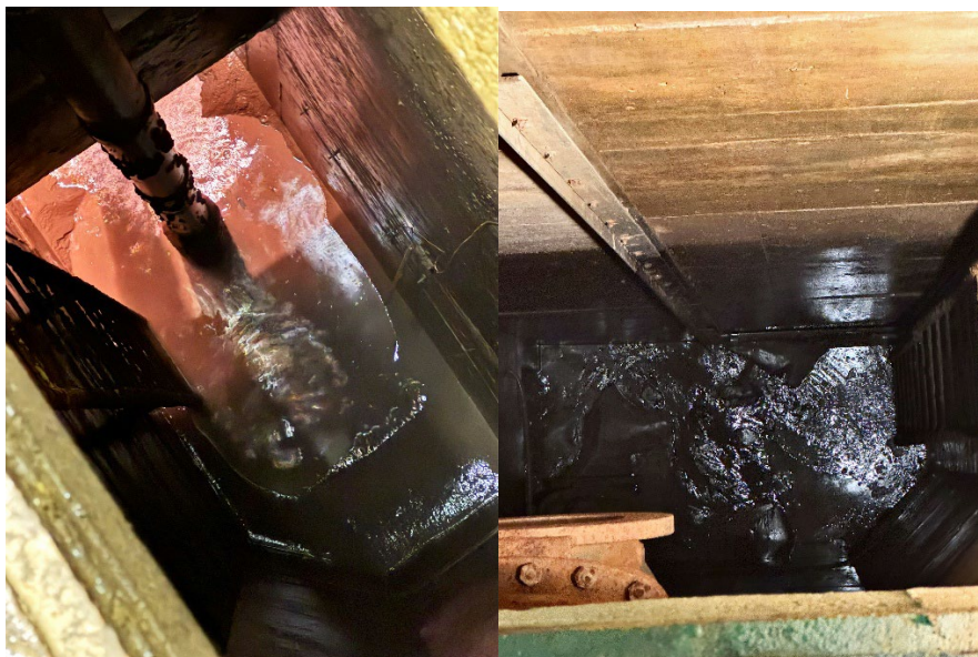
Filter 3 in the water plant under maintenance
