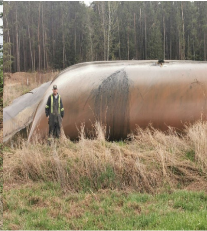
Geo tube for cell 1 east sludge
