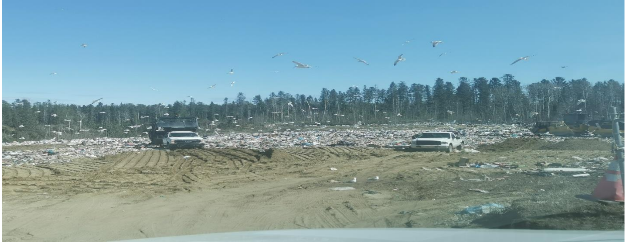
Landfill spring cover work starting
