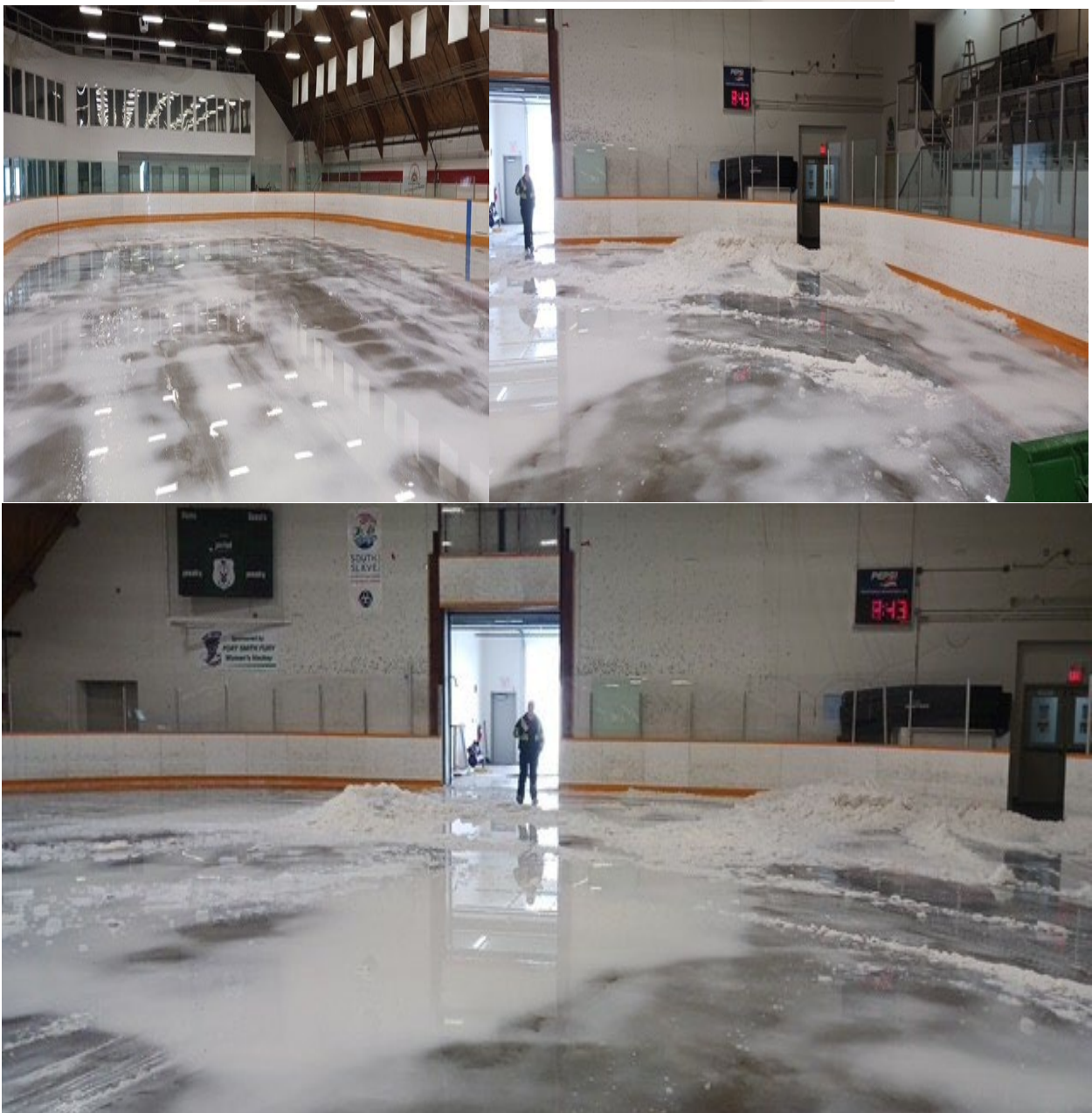
Removing arena ice
