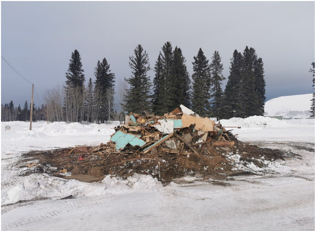
Old Firehall has been demolished.
